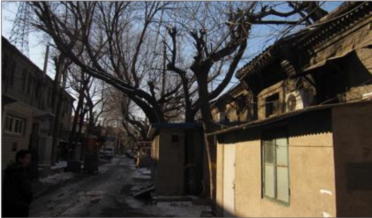
Figure 2: Kuei Chia Chang, looking west, with additions attached to the original building walls, January 2010 (courtesy: Jo Lusby)
